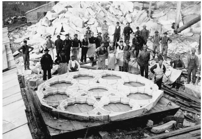
Workers on rose window
